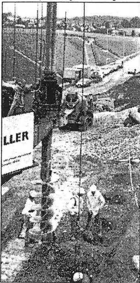
Contractors pile-drilling near the bridge
